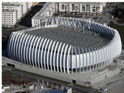
Figure 6 Sports hall "Arena Zagreb"
