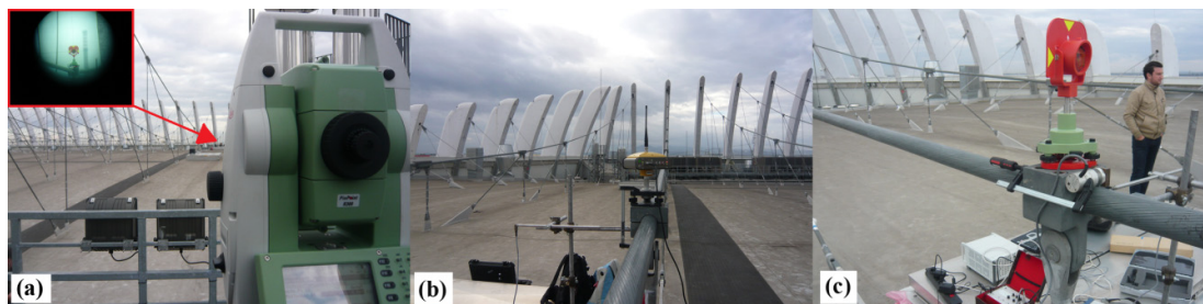
Figure 8 RTS (a), GNSS rover and LVDT sensor (b), prism and accelerometer mounted on the main cable (c)
