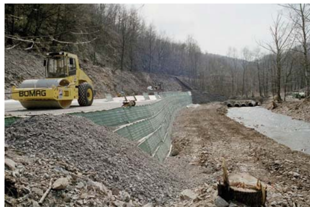
Fig. 19. Geogrid-reinforced railway embankment
