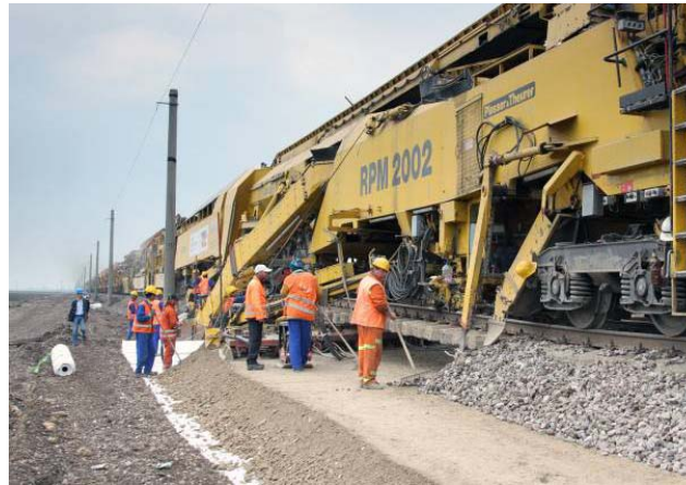
Fig. 10. Installation of FPL and Ballast on Secutex ® 251 GRK 4 and Secugrid ® 30/30 Q1
