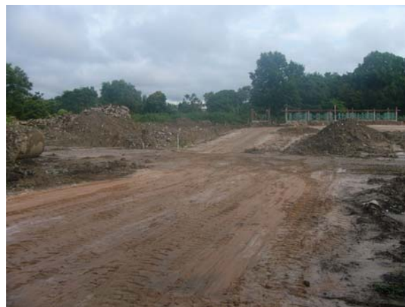
Fig. 17. Limited rutting of the reinforced courses
