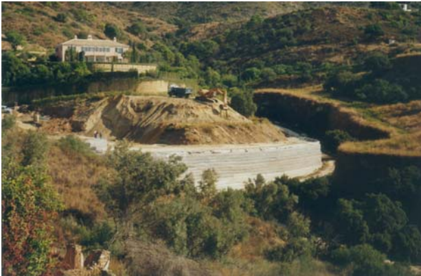
Fig. 22. Construction of the base wall (10 m high)
