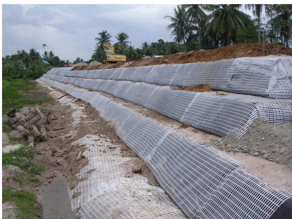
Fig. 14. Reinforced slope during construction
