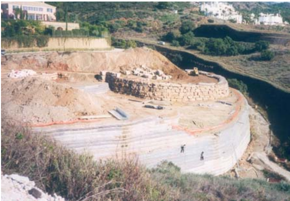
Fig. 24. Installation of a natural stone block facing for the semi-circle geogrid reinforced soil structure (August 2003)
