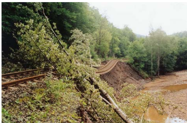
Fig. 18. Collapsed railway embankment after flooding
