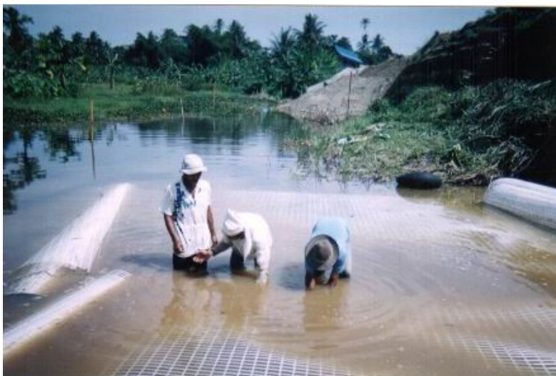
Fig. 13. Extreme soil conditions on the site
