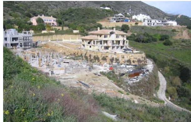
Fig. 25. Villa constructed on reinforced soil structure (May 2006)
