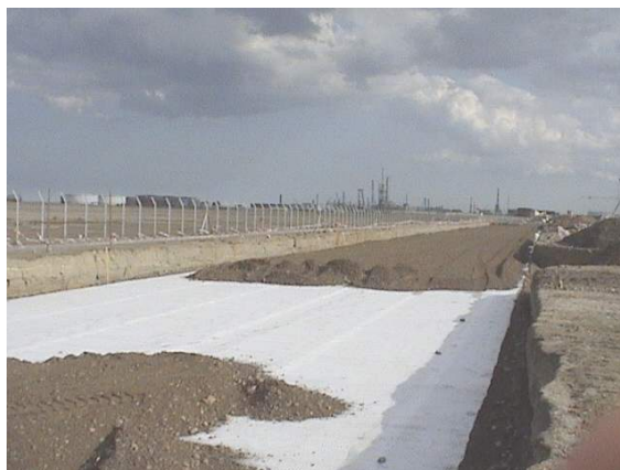
Fig. 12. Installation of Secugrid ® base course reinforcement
