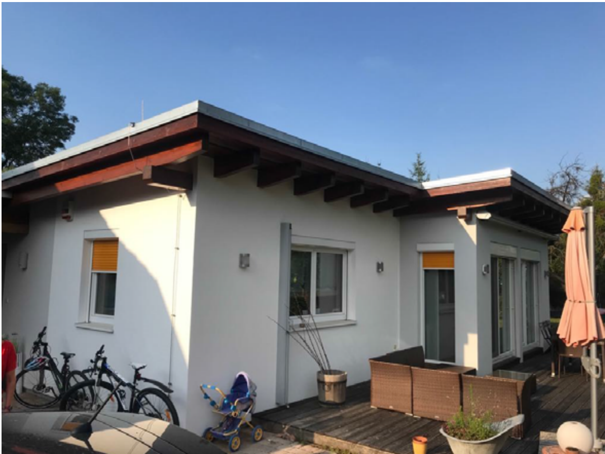
Figure 1: The evaluated building
