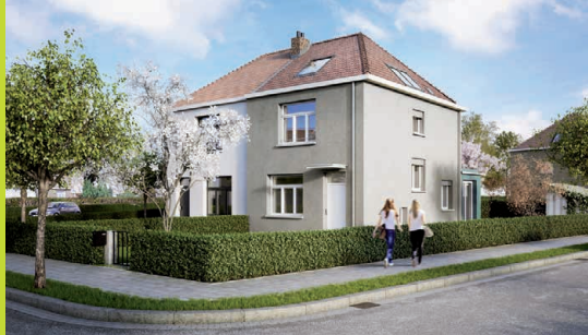
RenovActive House – Brusel
