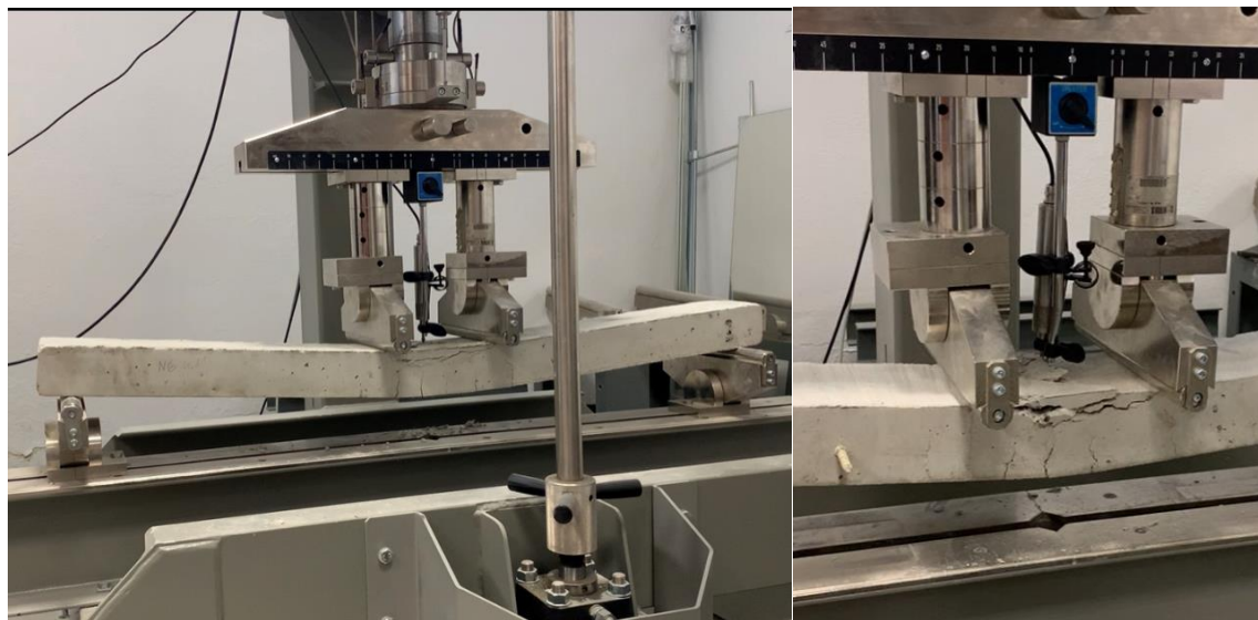
Figure 3-4 The failure of the concrete crushing during a four-point test
