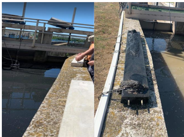
Figure 3-11 Beams before and after being placed into the inflow channel
