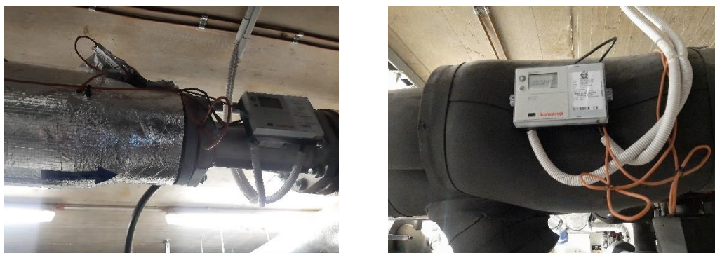
Fig. 6.4 Calorimetric heat and cold generation counter in Ecopoint 2
