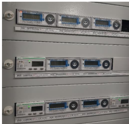
Fig. 6.3 Electrometer Schneider Electric in Ecopoint 2
