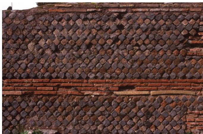
Obr. 3-2-20. Opus Mixtum zhotovené z opus reticulatum a opus testaceum v Ostii.
