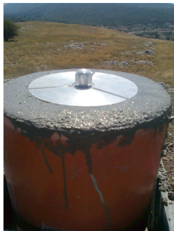
Figure 5 Pillar for horizontal network of hydropower system "Dabar" in construction
