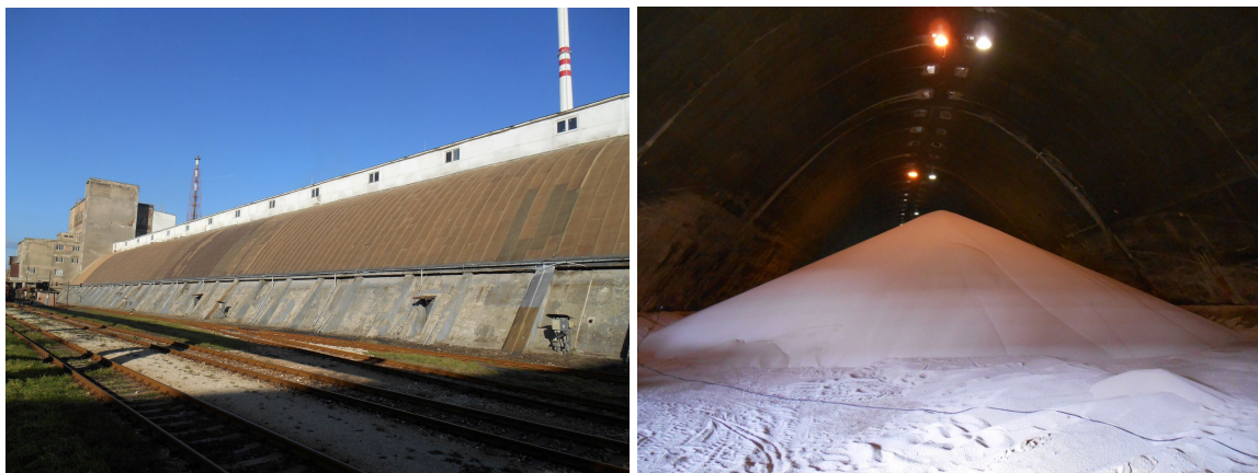
Figure 1 The construction of the warehouse
