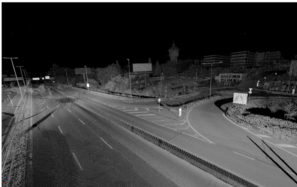
Figure 2 Basic output: 3D point clouds with details of road and surroundings
