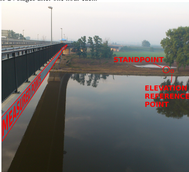
Figure 2 Measured points on the side of the bridge, standpoint and reference point
