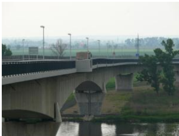
Figure 1c The bridge near Litoměřice
