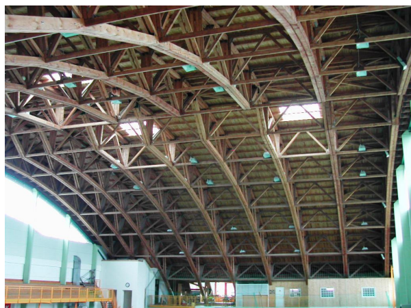
Figure 3 Roof after its completion
