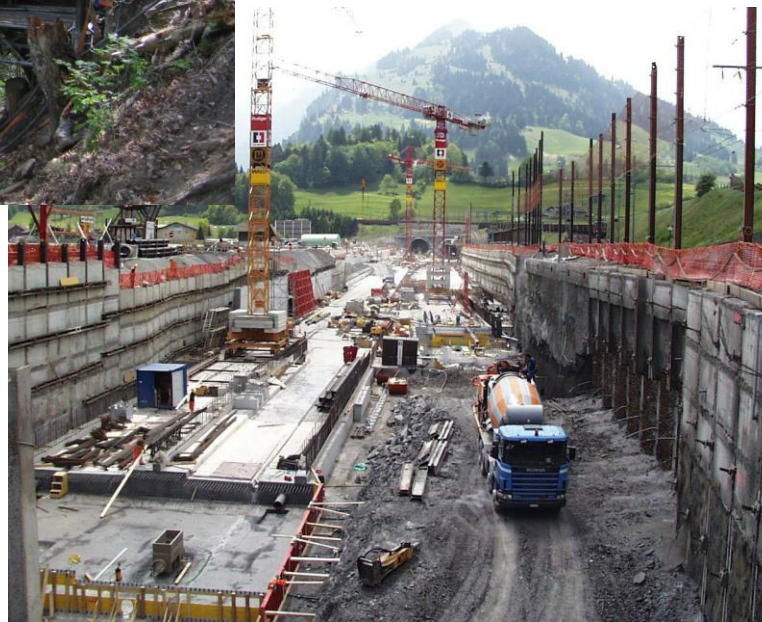
Deep excavation Alptransit Lötschberg
