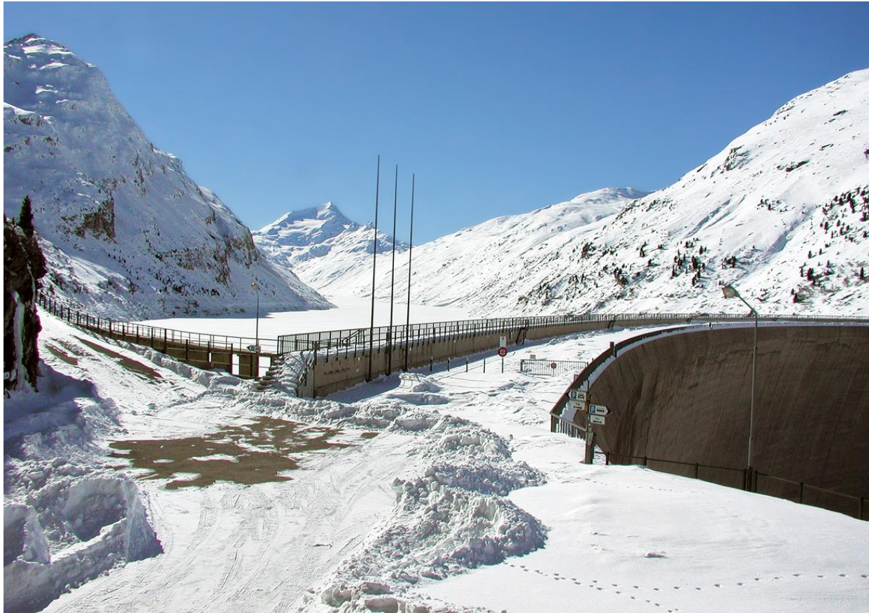
Concrete arch dam Valle di Lei, Switzerland
