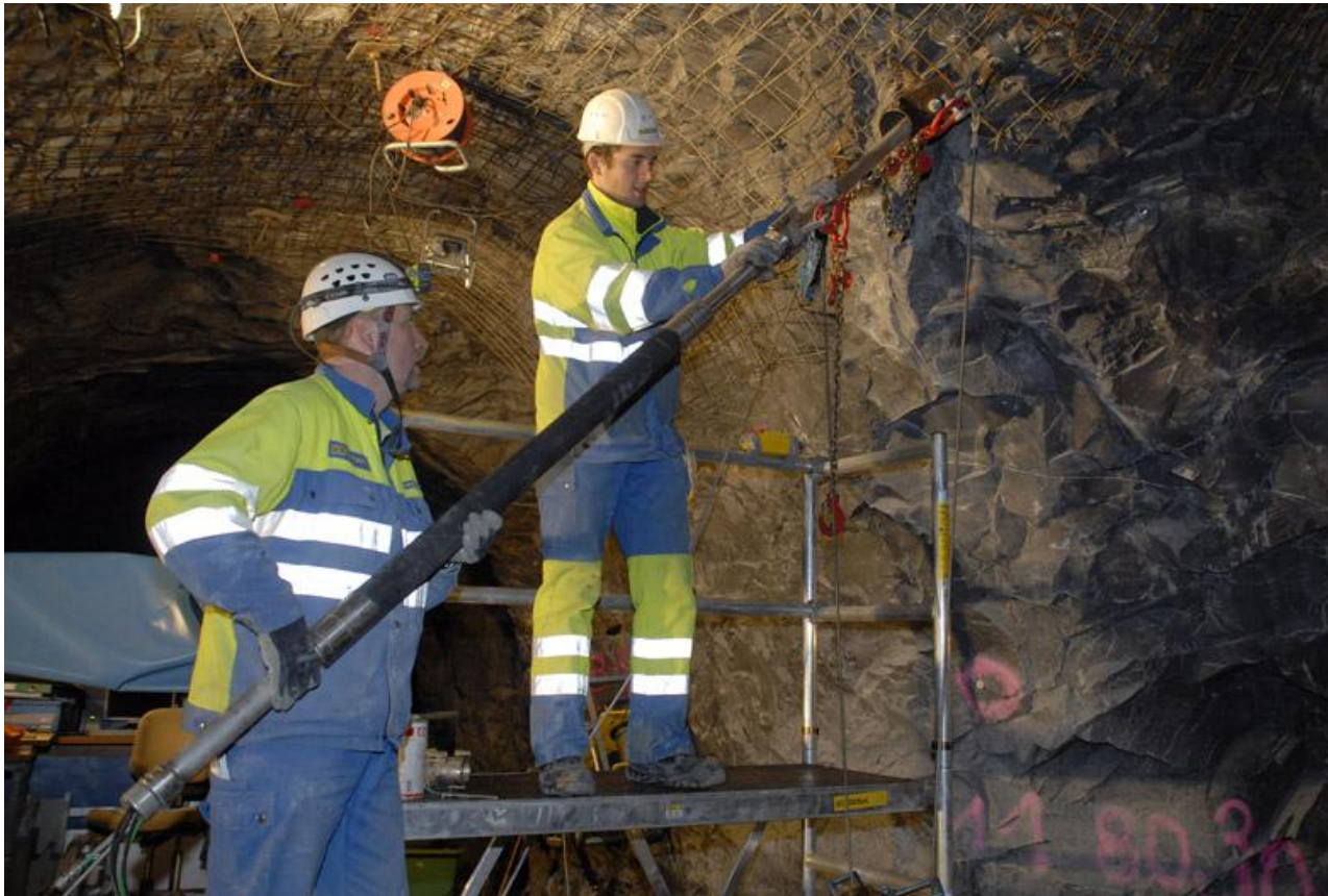
Hydro tests underground to explore ground water conditions for the turbine cavern
