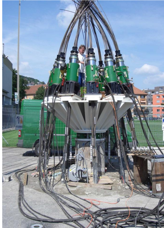
Stadium Hardturm, Zürich, pile diameter 1.20m length 15.0 m measurement of strain distribution with Sliding Micrometer
